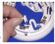
hole on the detector cover to depress the locking device.
